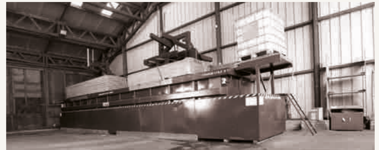
Class 2 treatment tank - Bouguenais site (44)
