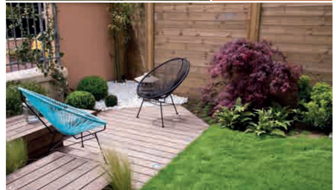
1, 2 and 3. Green treatment / 4. Brown treatment 1, 2, 3, 4. Blades 28x135, posts 45x90, finishing board 28x70
