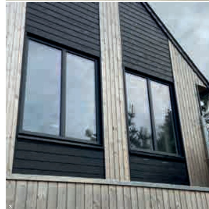
1 and 2 Cladding just installed / 3 and 4. Cladding 1 year after installation
